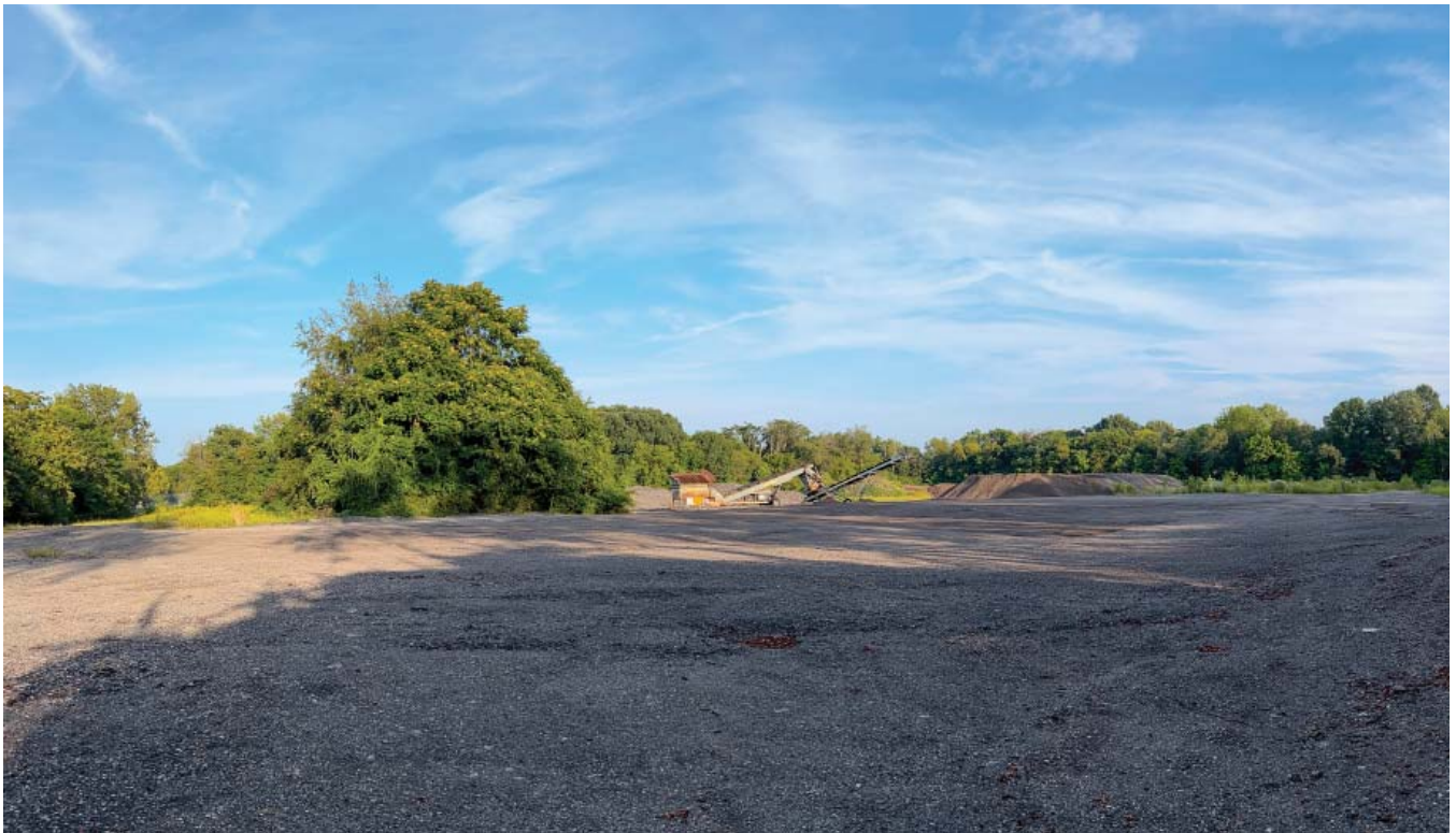
Figure 59. Southerly view of the Southeast field's asphalt operation
