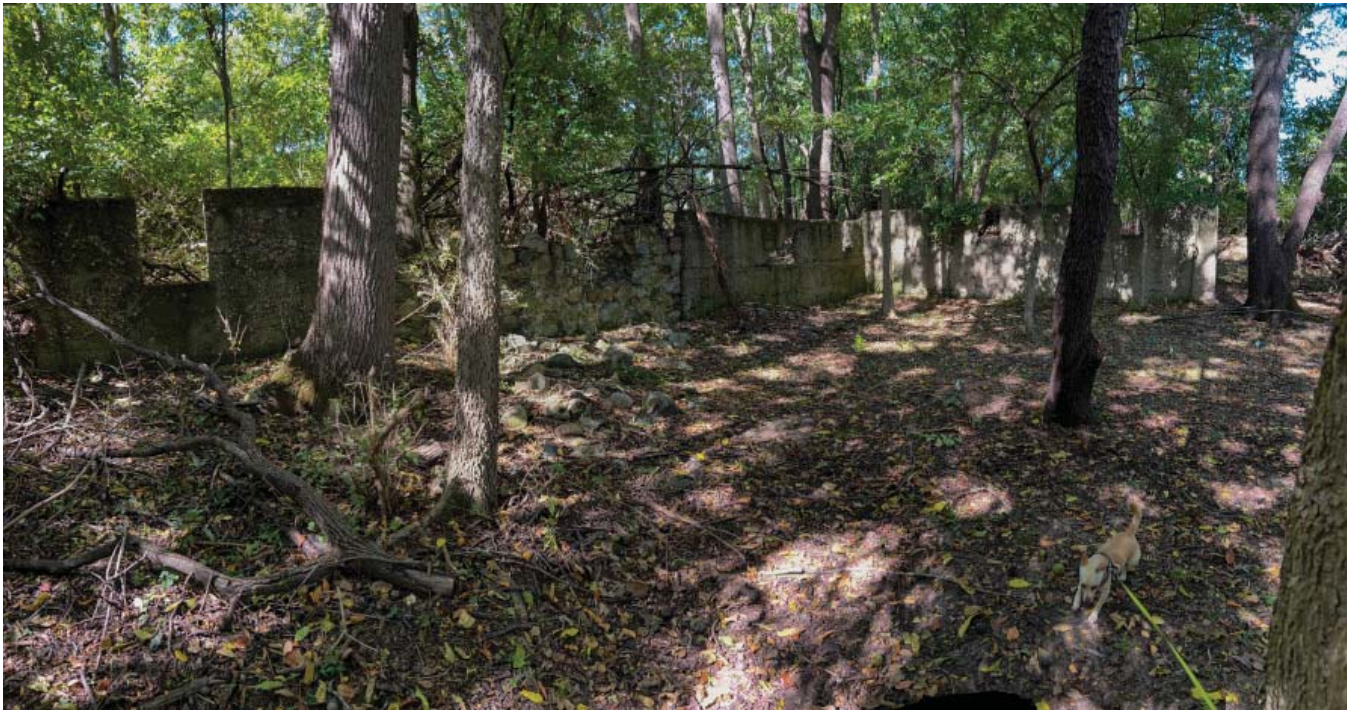
Figure 85. The remains of the foundation of a barn in the Early Successional Woods showing a combination of concrete and field stone construction.
