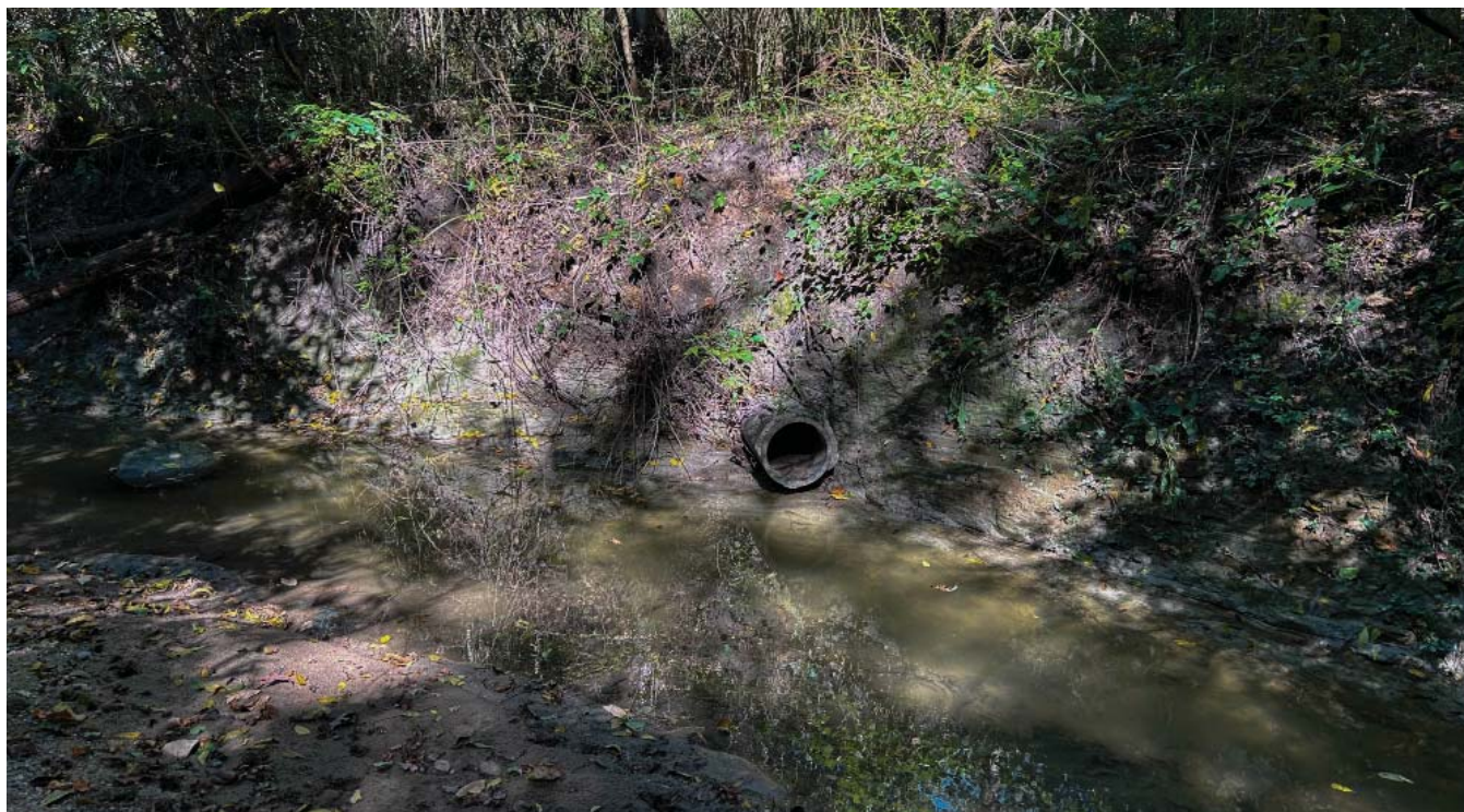
Figure 88. One of several agricultural drainage pipes in the Ravine
