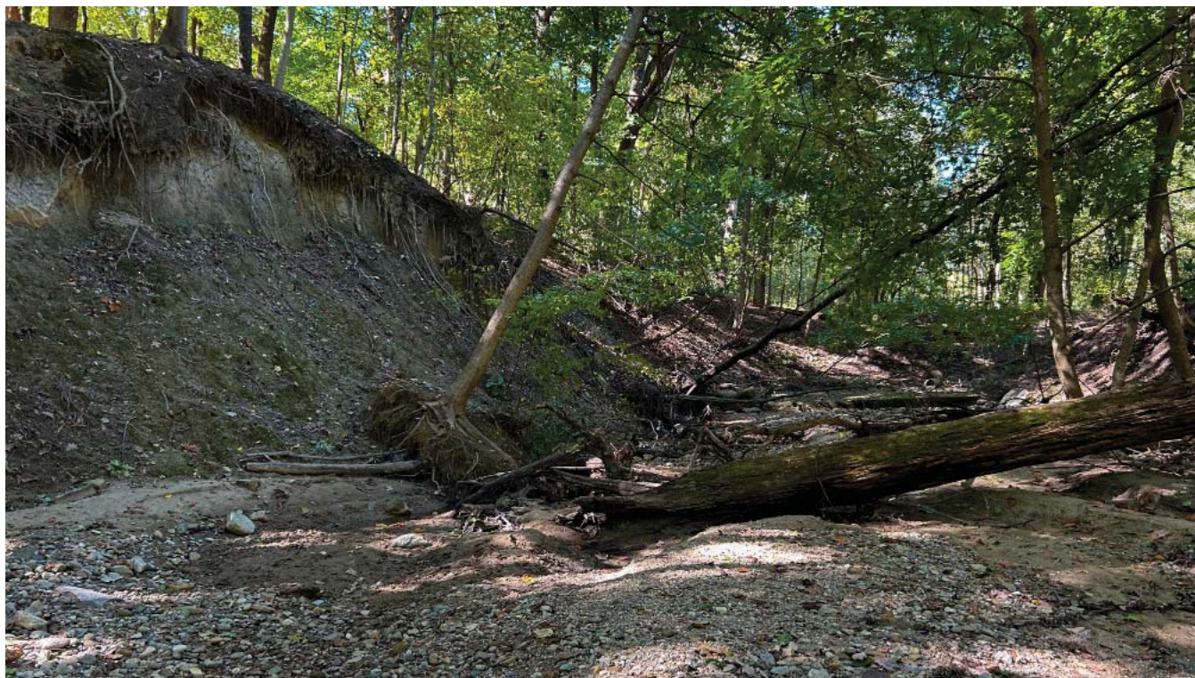
Figure 87. An area of the Ravine with undercut banks likely due to increased stormwater discharge
