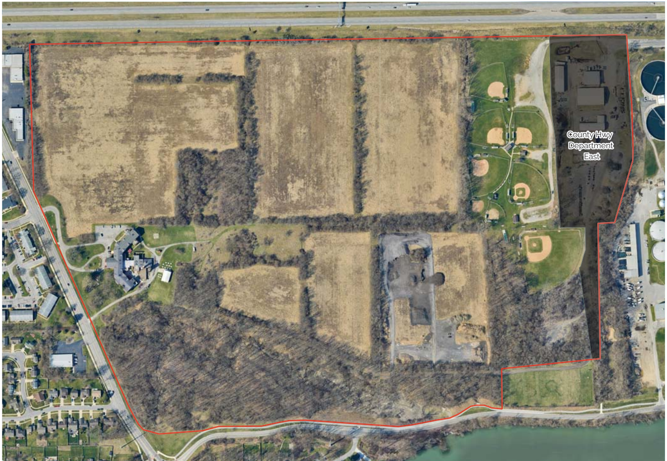
Figure 79. The County Highway Department East property and drive on the far eastern edge of the Portage Manor campus
